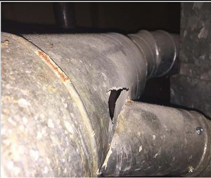
Image information: Opening in the furnace/water heater chimney.
