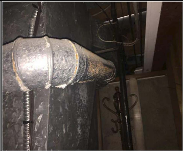
Image information: Rusting and moisture stains on the furnace chimney.
